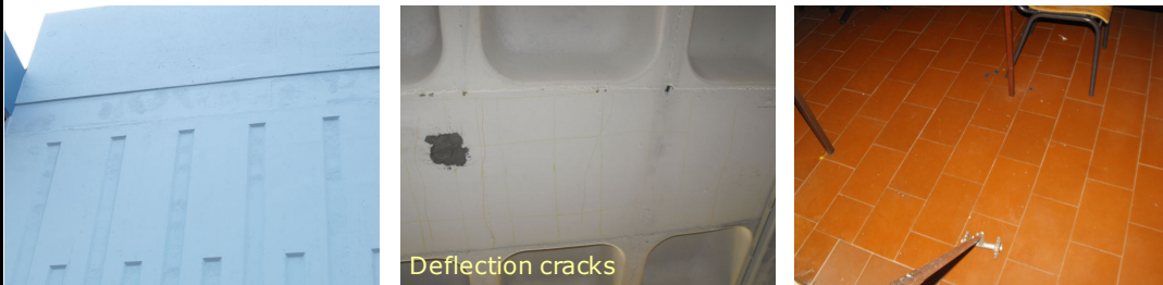
CONCRETE DURABILITY INSPECTION AND TESTING AT SCHOOL BUILDINGS STRUCTURE
