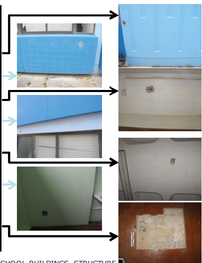
CONCRETE DURABILITY INSPECTION AND TESTING AT SCHOOL BUILDINGS STRUCTURE
